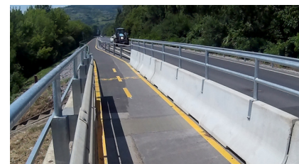
The installed POLYFLEX®ADVANCED joint on the south abutment of the bridge
