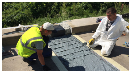
Casting of the POLYFLEX®ADVANCED PU joint
