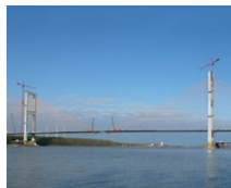
Audubon Bridge (USA)
