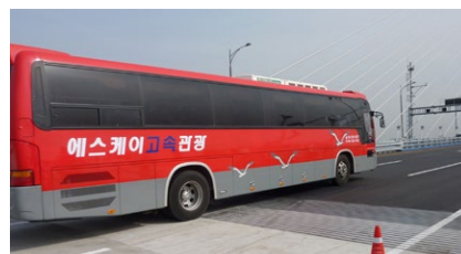
A mageba modular expansion joint in service
