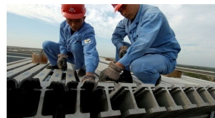
TENSA®MODULAR expansion joint type LR24 ready for installation
