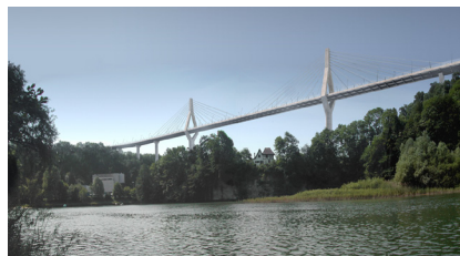
The Poya Bridge across the Sarine River
