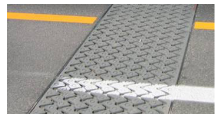
Installed modular expansion joint with noise reducing sinusplates
