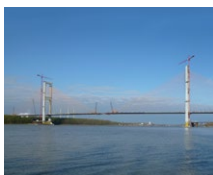
Audubon Bridge (USA)
