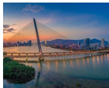
Tran Thi Ly Bridge (VN)
