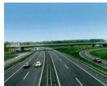
Freeway overpass Moosgasse, (CH)
