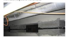
A TENSA®SLIDE sliding plate expansion joint bridges the gap along the building's foundations
