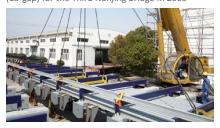
TENSA®MODULAR expansion joints (20-gap) as installed on the Second Nanjing Bridge in 2000
