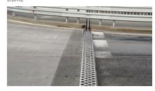
Close view of the of the supplied TENSA®GRIP RS-LS joint
