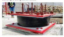
A RESTON®SLIDER bearing as installed to support part of the building's superstructure
