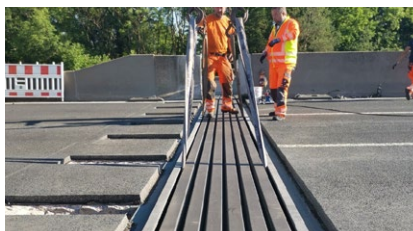
Lifting one of the new modular joints in place
