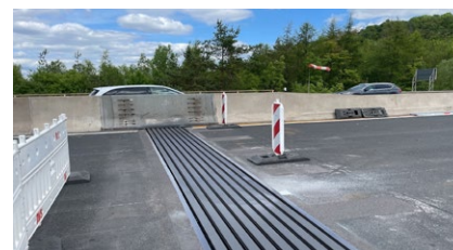
A replaced TENSA®MODULAR LR9 joint after installation
