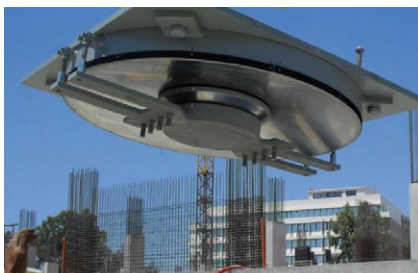
Curved surface slider bearings
