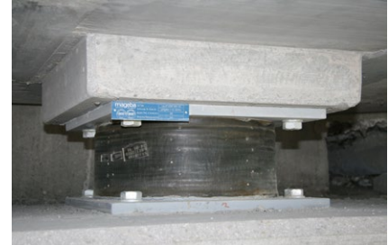
High damping rubber bearings
