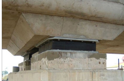
Lead rubber bearings
