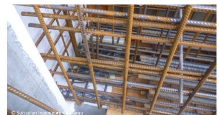
LASTO®FLONBLOCK under reinforcement cage, later sliding wall
