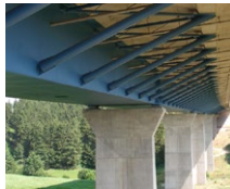
Steinbachtal Bridge (DE)
