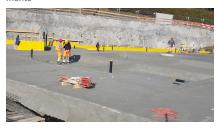
VIBRAX®DAMP elastomer mats during installation on the construction site
