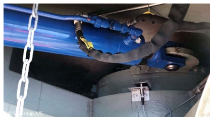
New mageba RESTON®SPHERICAL bearing after installation, alongside the bridge hydraulics
