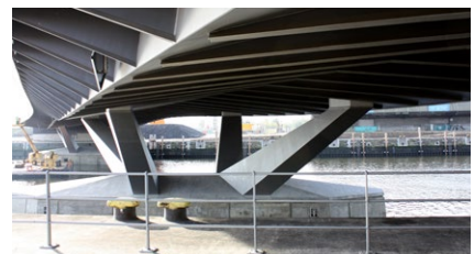
The bridge's V-beam is supported by elastomeric and spherical bearings
