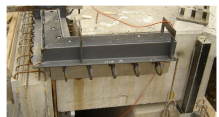
The sliding plate construction is fixed to the bridge substructure
