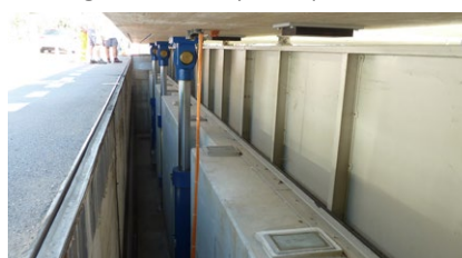
The specially designed elastomeric bearings and the lifting device with 4 hydraulic pistons
