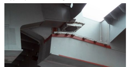
Support points of the finger lock
