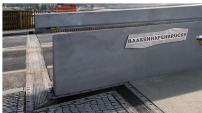
The mat joints are shaped to fit the given vertical and horizontal bends of the Baakenhafen Bridge
