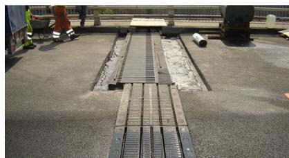
A TENSA®FLEX Type RC400 expansion joint during installation on first side of deck.
