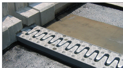
An installed TENSA®RSFD cantilever finger joint prior to placing of asphalt road surfacing
