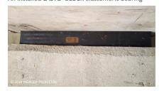
Horizontally and vertically oriented bearings as installed at end of deck section
