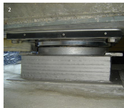
1 KE bearing showing dust protection apron and movement indicator, ready for installation 2 Installed KA bearing with dust protection apron temporarily removed
