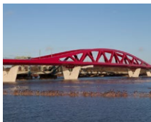
Ijssel Bridge (NL)
