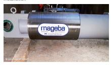
Installation of RESTON®SA shock absorbers (fluid viscous dampers) at one end of the bridge
