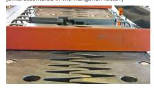
TENSA®FINGER joint were built in sections leaving space for the new railway tracks
