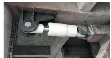
A RESTON®SA shock absorber after installation
