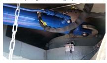
Rotation caused during bridge opening is facilitated by the RESTON®SPHERICAL bearing
