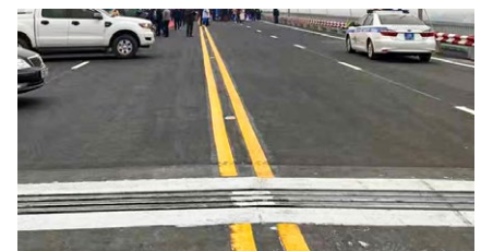
An installed TENSA®MODULAR LR4 joint
