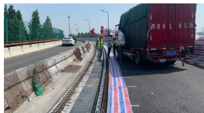
Preparation of the substructure
