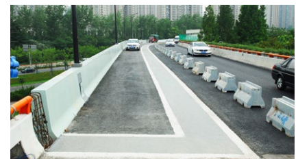
TENSA®POLYFLEX®ADVANCED PU joint after installation
