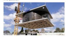
Installation of a LASTO®LRB lead rubber bearing to the building
