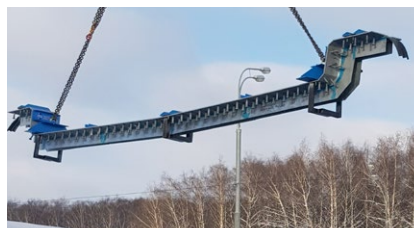
A TENSA®RAIL RSU joint during unloading on site
