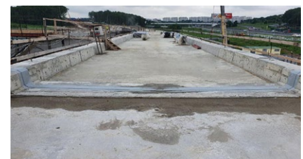
TENSA®RAIL RSU installed on site
