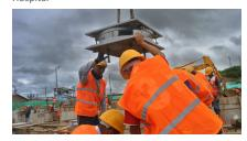
Precise positioning and levelling of a RESTON®PENDULUM seismic isolator
