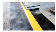
A prefabricated joint with a non-slip cover plate in the waiting hall of the railway station
