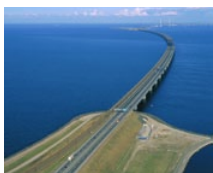
Storebaelt West Bridge (DK)
