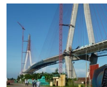
Can Tho Bridge (VN)
