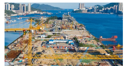
The Kai Tak Cruise Terminal during construction
