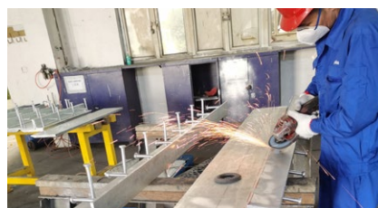
Joints in production
