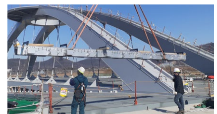
Lifting of a TENSA®MODULAR LR3 expansion joint on site
