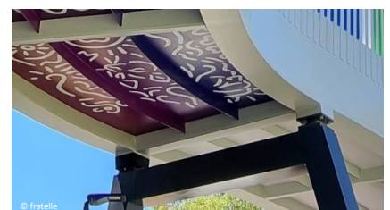
RESTON®POT HP bearings installed on the pylons of the bridge
