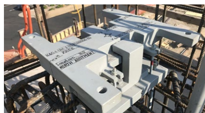
Installation of a spherical bearing at Location B2
