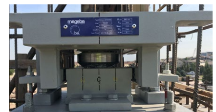
A guided sliding uplift type of spherical bearing at Location B1
