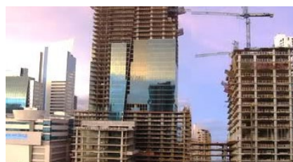
Construction of the Plaza
