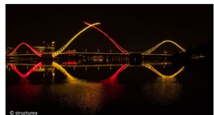
Night view of the Swan River Pedestrian Bridge
