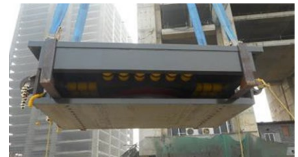
Installation of the ERADIQUAKE® seismic isolator
