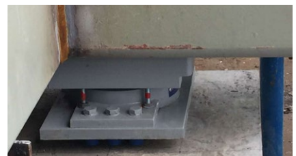
An installed RESTON®POT bearing
