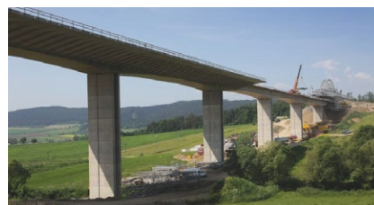
Impression from the construction site
