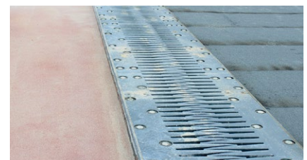
Close-up picture of an installed TENSA®FINGER cantilever finger joint
