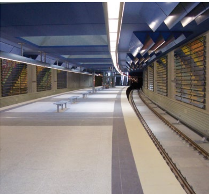
Hamburg airport, underground
