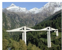
Ganter Bridge (CH)
