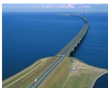
Storebaelt West Bridge (DK)
