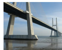
Vasco da Gama Bridge (PT)
