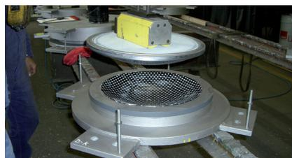
Installation of two TENSA®MODULAR expansion joints, end to end, at one bridge axis.
