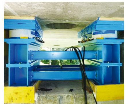
Lifting and lateral adjustment works
