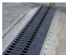
Sliding finger joints
