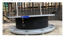
A pair of LASTO®HDRB isolators as installed on site
