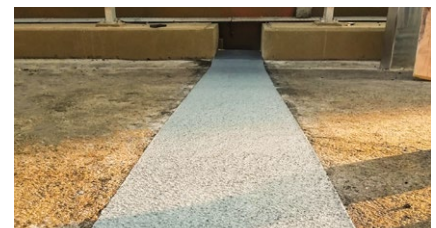
TENSA®POLYFLEX® joint after installation
