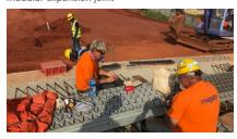
The sinus plates will reduce noise from overpassing traffic by up to 80%
