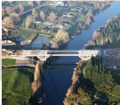
Waikato River Bridge | New Zealand
