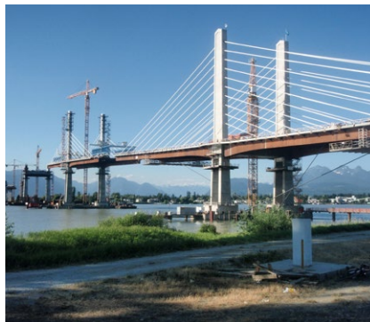
Golden Ears Bridge | Canada
