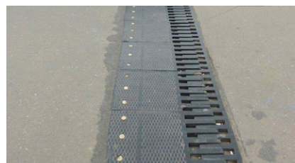
TENSA®FLEX RC200 joint installed in 2001
