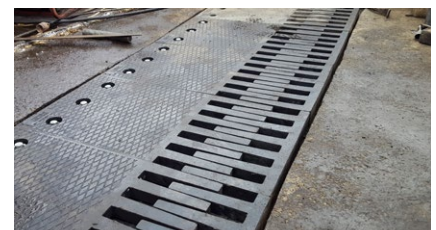
TENSA®FLEX RC200 joint installation in 2015
