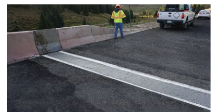
The completed joint high in the Rocky Mountains of Colorado
