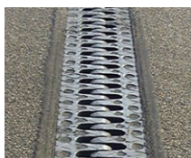
Cantilever finger joints
