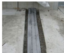
Joint prior to concreting
